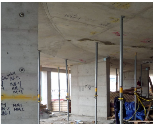
Figure 17: View of transition from 9" slab to 18.5" slab
