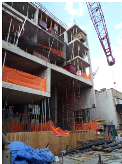
Figure 18: Cantilevered slab as part of balcony system
